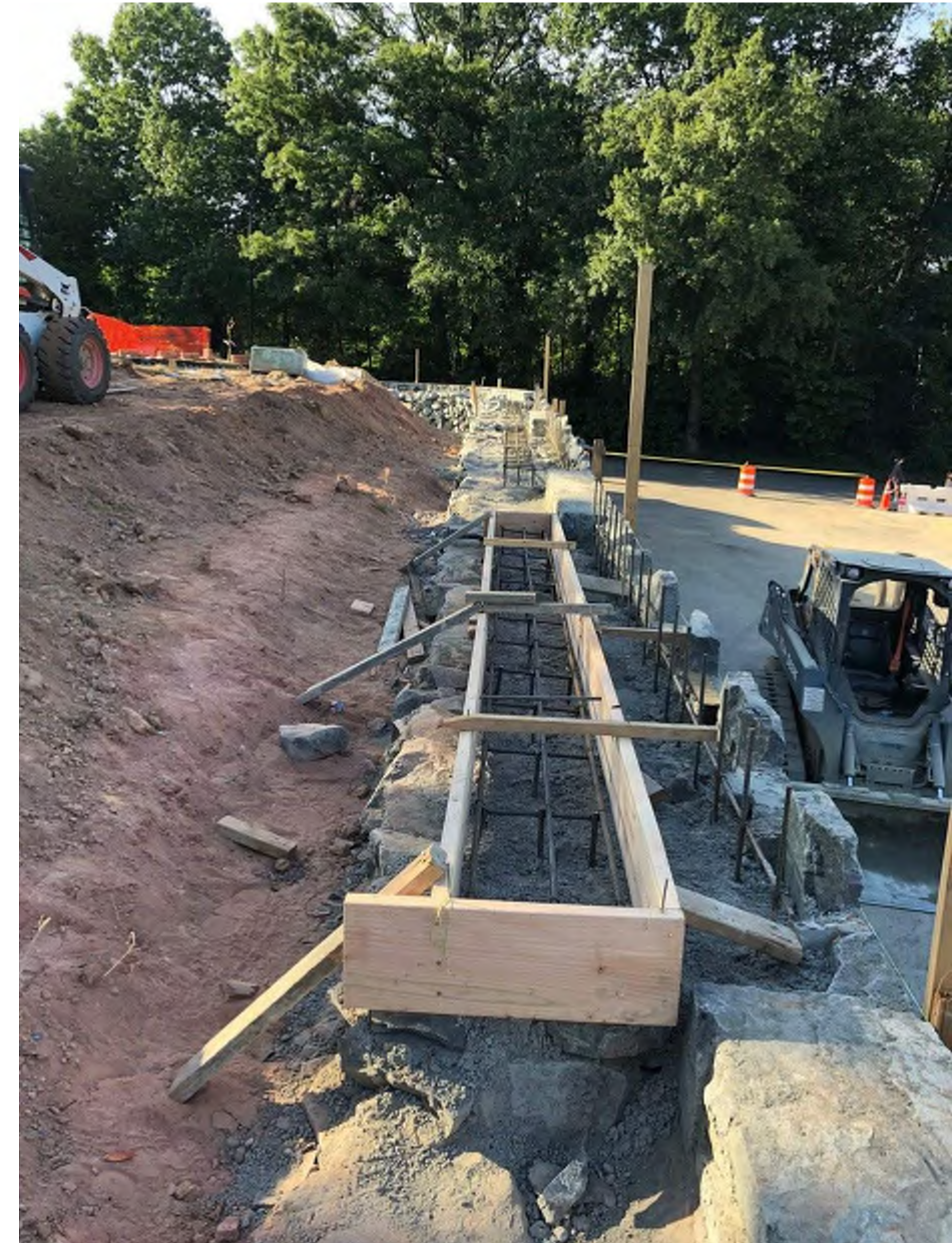
The foundations for the first phase columbaria are integrated with the parking lot-facing new stone retaining wall
