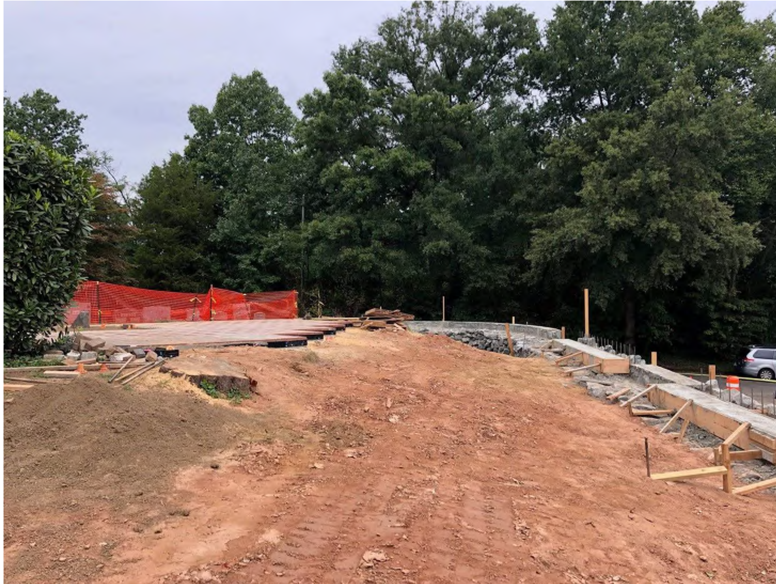
The foundations for the first phase columbaria are integrated with the parking lot-facing new stone retaining wall
